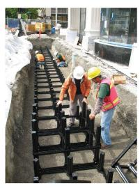
Silva Cell being installed on Fourth Avenue in Seattle in August 2009. Silva Cells support a tree by providing sufficient soil volume for the tree roots to expand within the modular system (below the pavement) and by reducing soil compaction.
